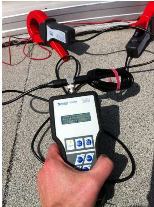
Illustration 07: Application of Ground-fault location kit
