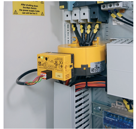
CTUB100 series measuring current transformer in the distribution units
